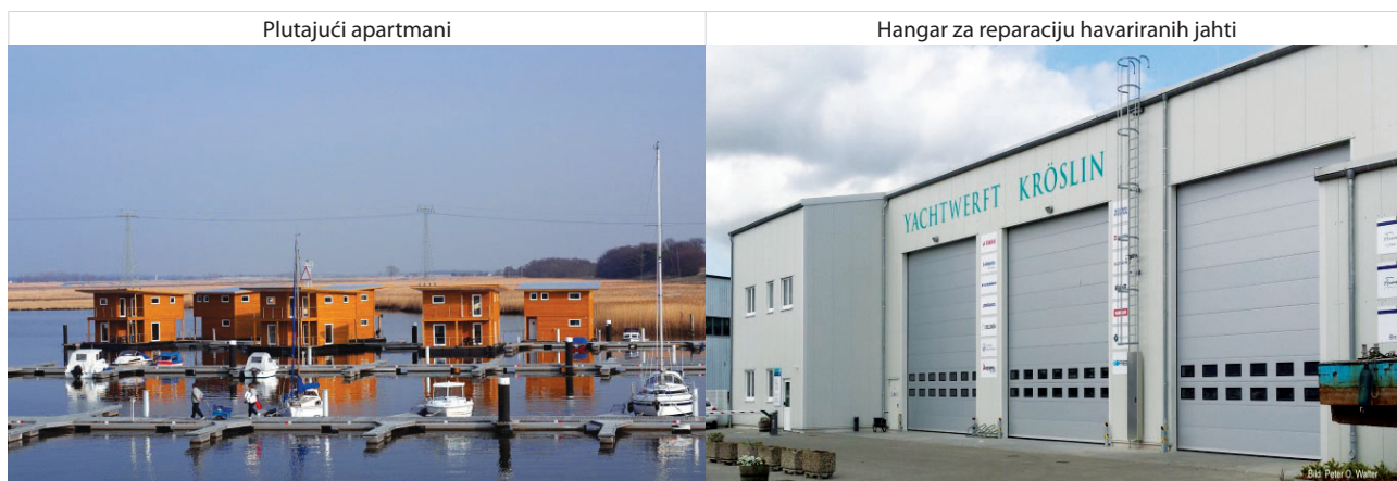
Slika 3. i 4. Plutajući apartmani; hangar za reparaciju havariranih jahti u marini Kröslin Figure 3 and 4 Floating apartments: containers for the repair of damaged yachts in Kröslin marina
