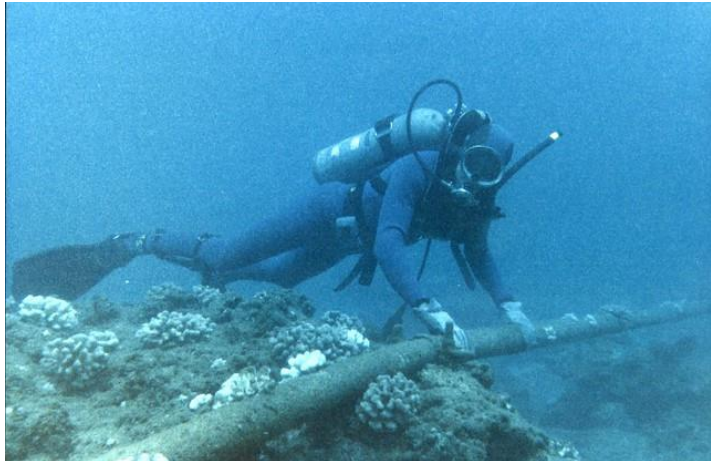
Picture 3. Diver during inspection of underwater cable Source: CTBTO Preparatory Commission (CC BY 2.0)
